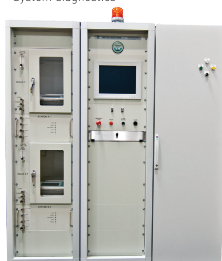
2 Station 2 Scale Cabinet
